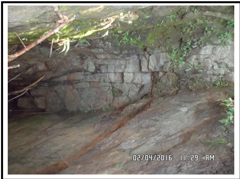
Plate – V: Adit and shaft structure in an abandoned graphite mine within the selected grid unit
