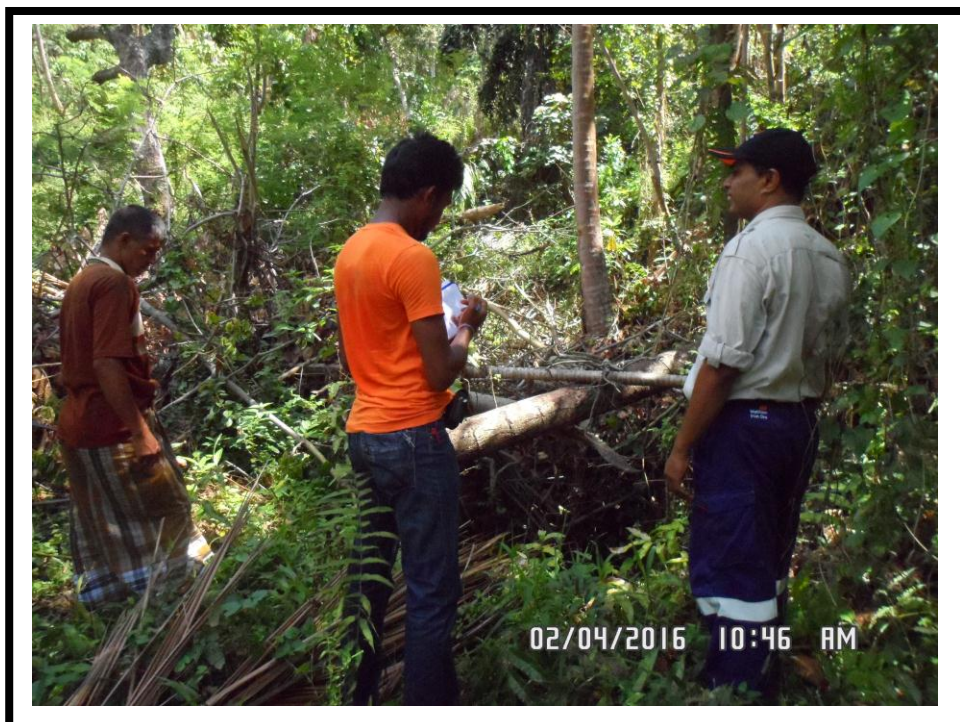
Plate – III: A partly filled shaft structure in an abandoned graphite mine within the selected grid unit
