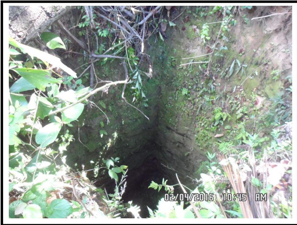
Plate – II: A partly filled shaft structure in an abandoned graphite mine within the selected grid unit
