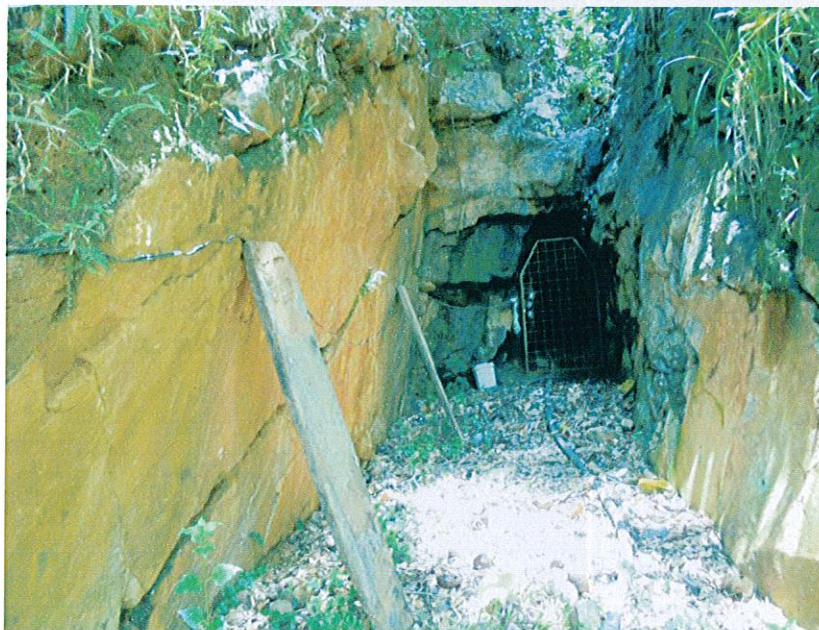
Plate (1.1): Main entrance of the mine, RS mines, Maduragoda, Dodamgaslanda.
